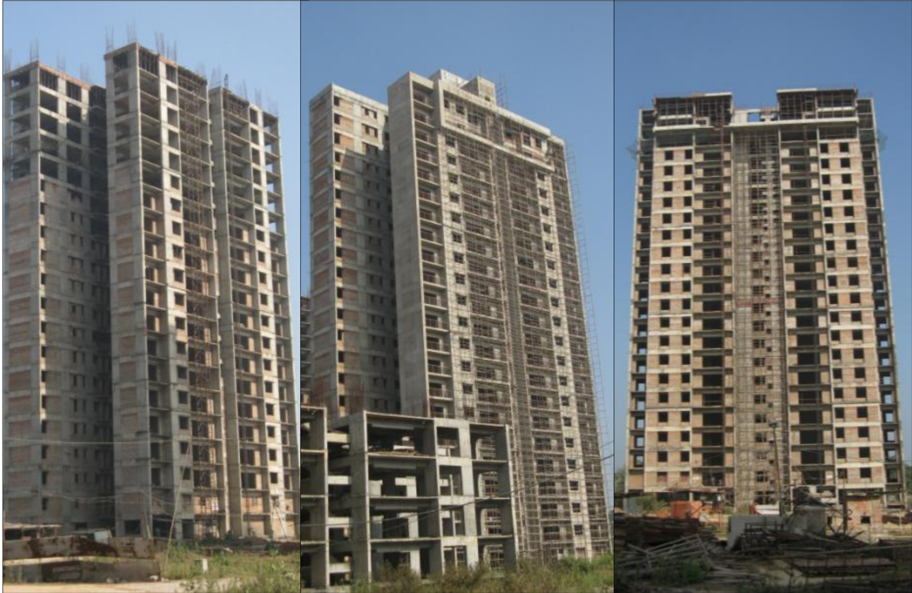
HARMONY, KOLKATA – Structure complete, internal work in progress
