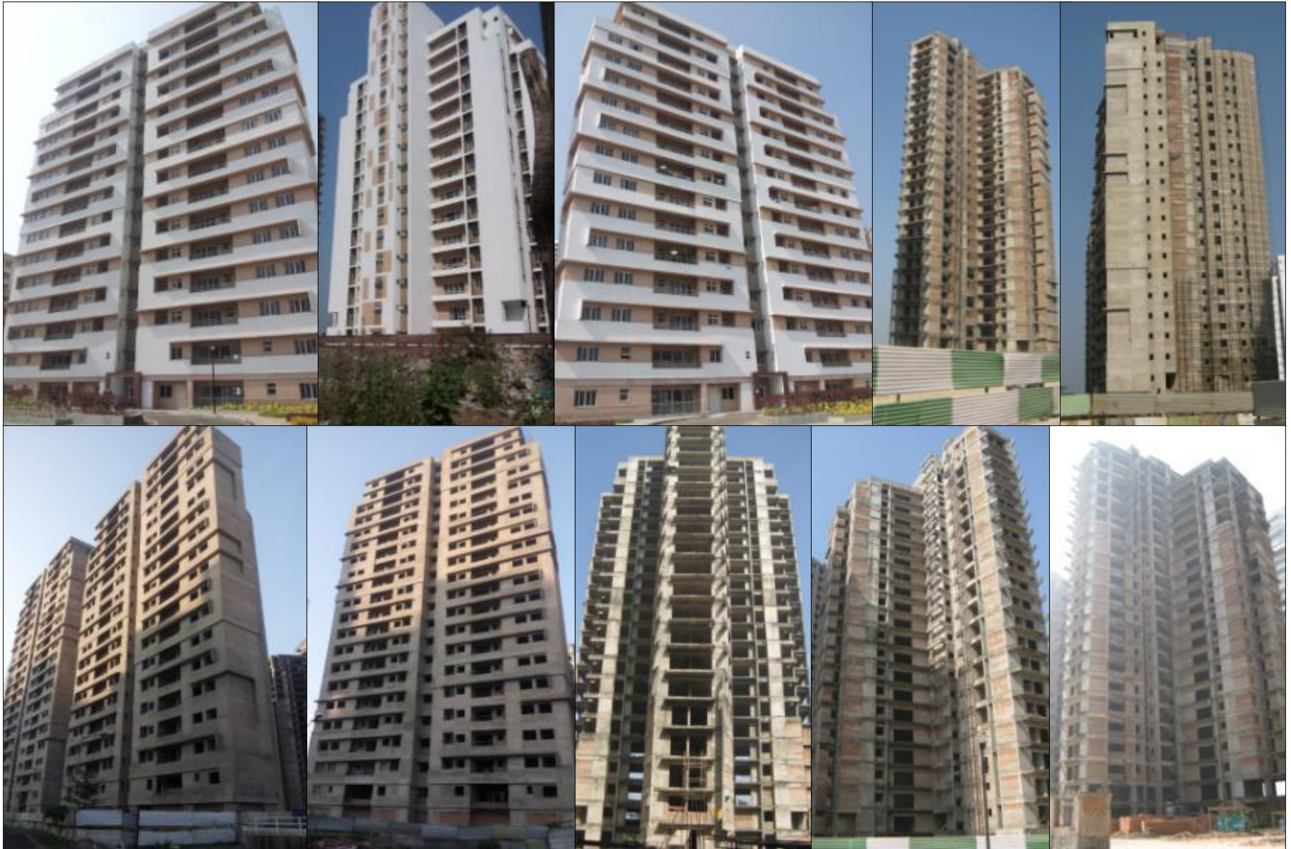
CASCADES, KOLKATA – Handover / Finishing in Progress
